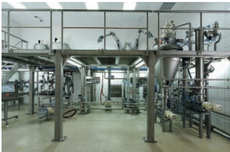
Continuous processing: Romaco FrymaKoruma's new plant for semi-solids such as toothpaste
