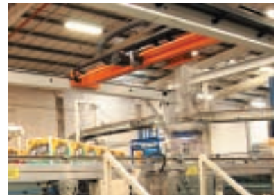
Automated palletising: Kuka software guides the KP Foods gantry system
